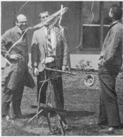
Mr. Knutson, Mr. Price, and Mr. Snyder inspect the "weird" welding" in the SE yard of the Junior High.
